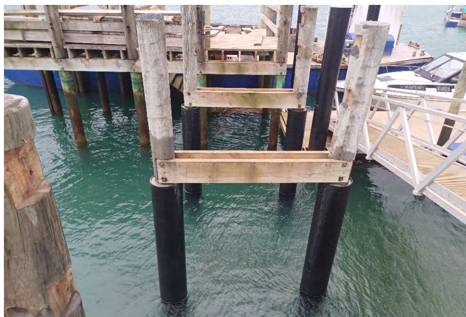
Timber piles with protective sleeves, Camp Bentzon, Kawau Island.
